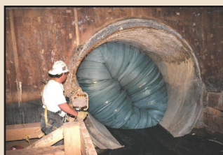
Inserted liner for repair
