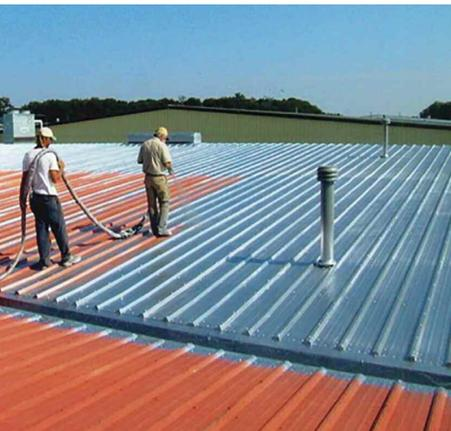
**DuraTite® 1175 and 1285** are high-solids, single-component, elastomeric, urethane coatings for new or existing roofing and waterproofing applications. Both offer superior impact and crack resistance while DuraTite 1285 also offers enhanced UV stability. DuraTite 1175 and 1285 can be applied in a wide range of ambient temperatures and humidity levels with a standard airless paint sprayer, brush roller, broom or squeegee.
