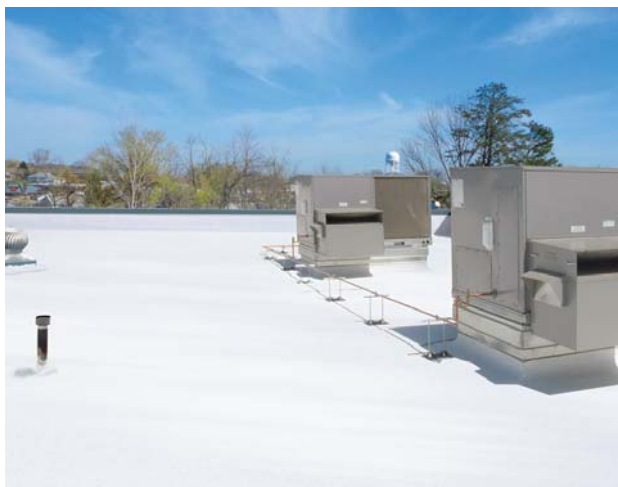
An excellent choice for roof restoration and renewal purposes
